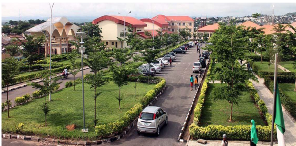
Figure 1: A Pictorial View of the Premises of Federal University Lokoja
